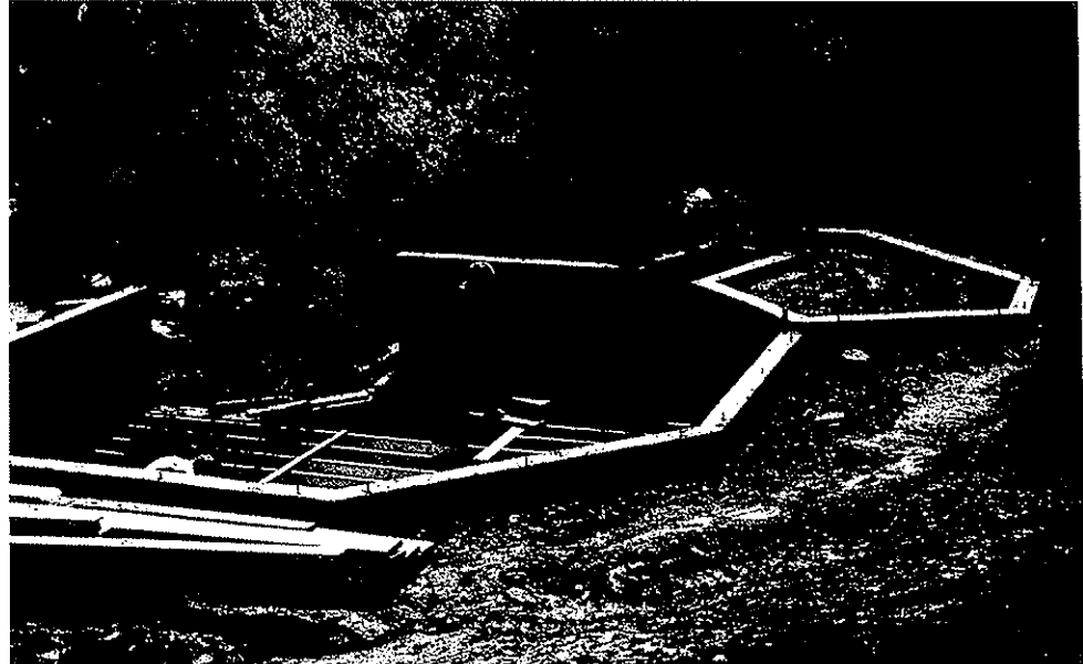
Poor soil conditions at the site dictated an engineered foundation. The octagonal wall is actually a poured-concrete grade beam supported by concrete caissons. The small polygon on the right is the foundation for the sunspace entry.
